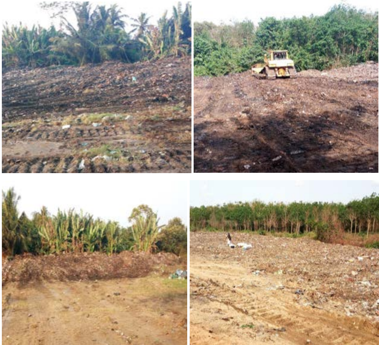
fig.3. After pushing at Nkroful and Ampain site
