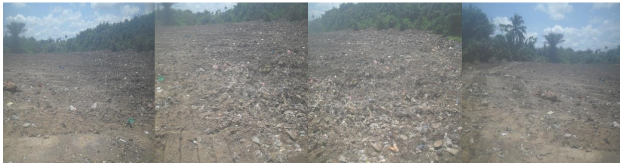
Fig. 5.After pushing at Ampain site
