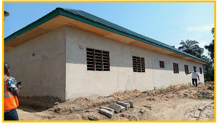
Construction of classroom block at Mandugbane
