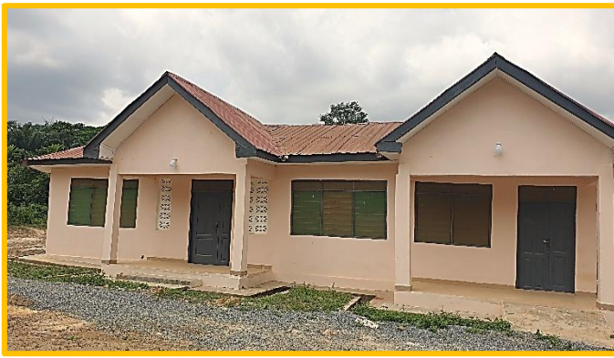
Front view of Aluku CHPS compound
