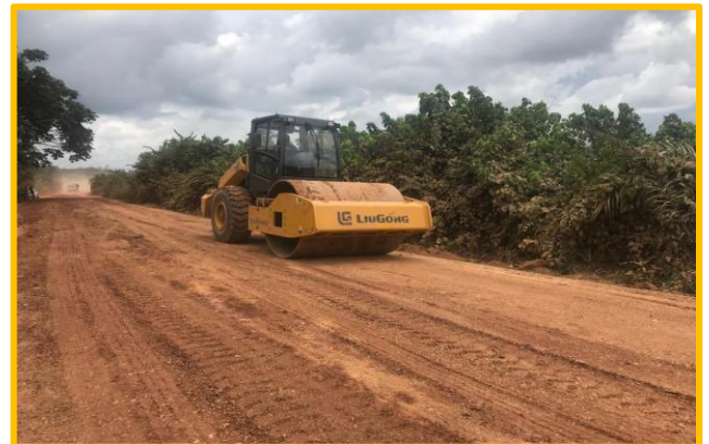
Grading of Salma/Aluku road
