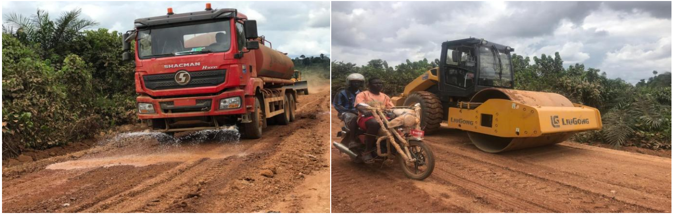
Reshaping of road using the DRIP machines
